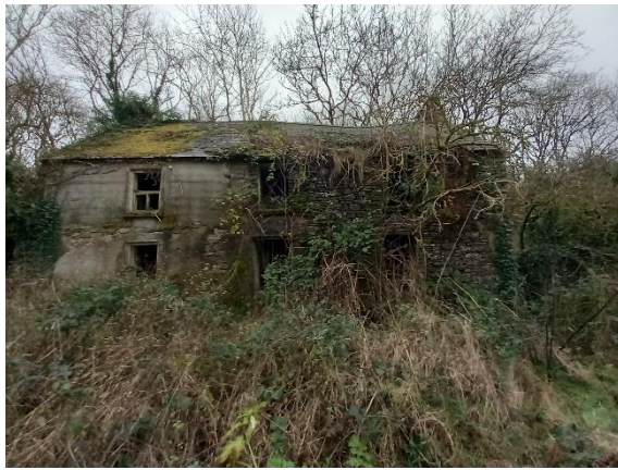
Building at B_06
