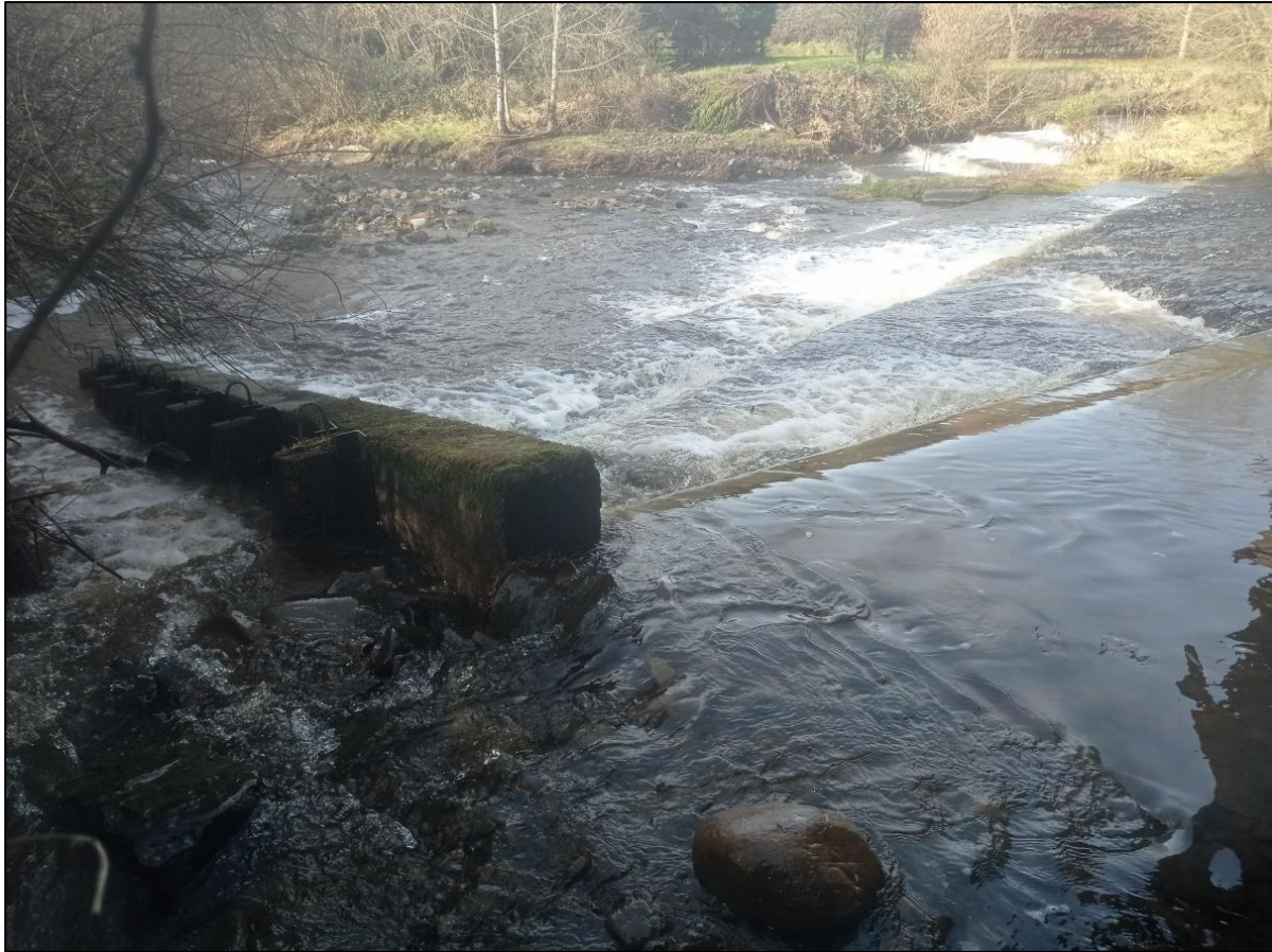
Plate 5.19: Fish Pass and Bridge Apron at Coan Bridge
