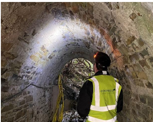
Inspection of Bridge 2.
