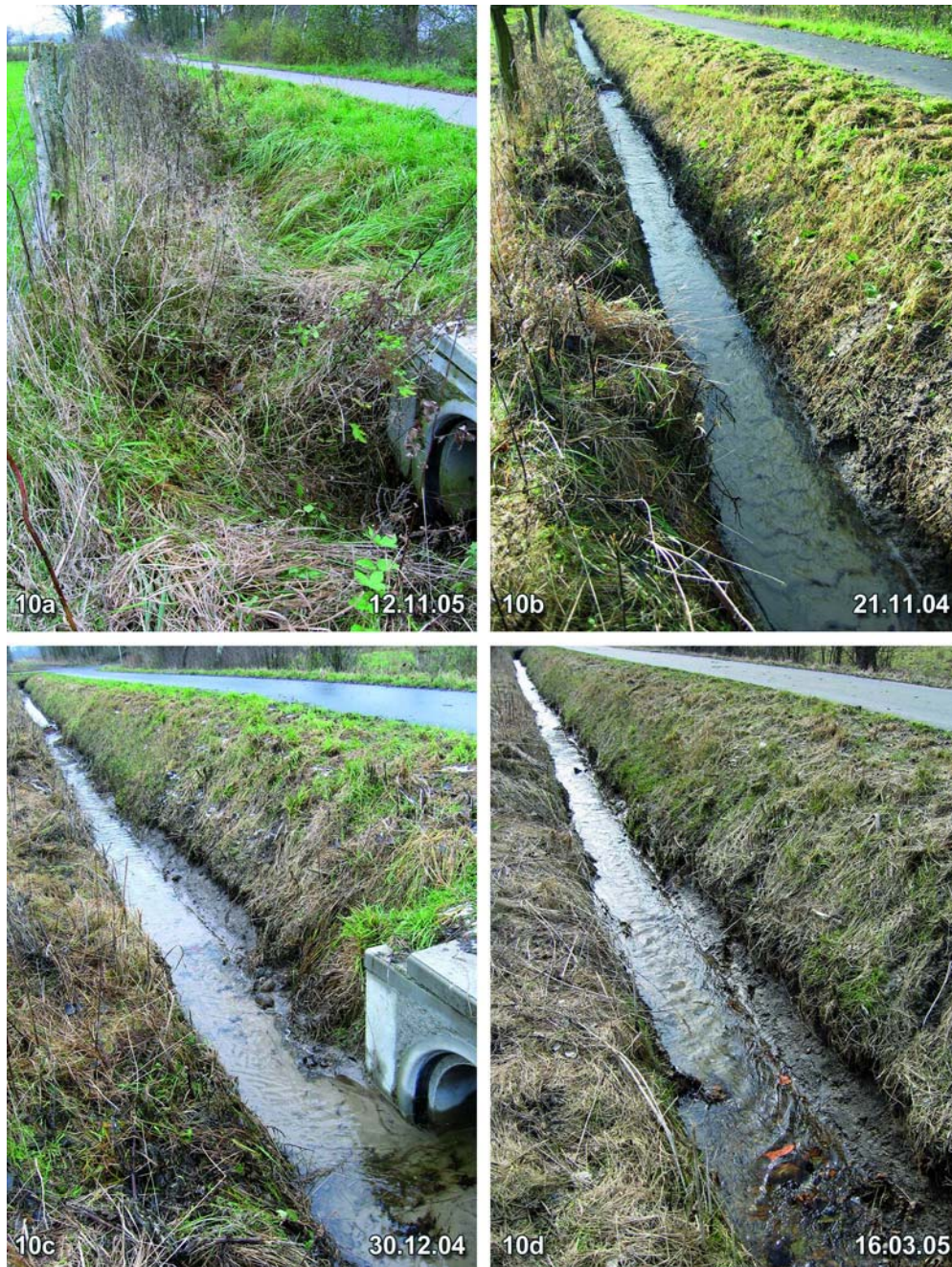
Fig. 10: Drainage ditch running parallel to the farm road. For position of the photographer see Fig. 8, top of the red arrow, view direction: sw.
