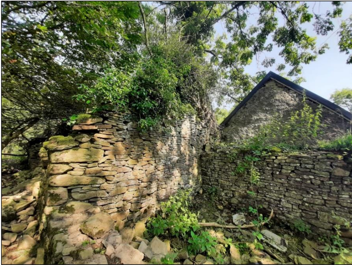
Plate 5.12: Stone Walls and Other Stonework (BL1)
