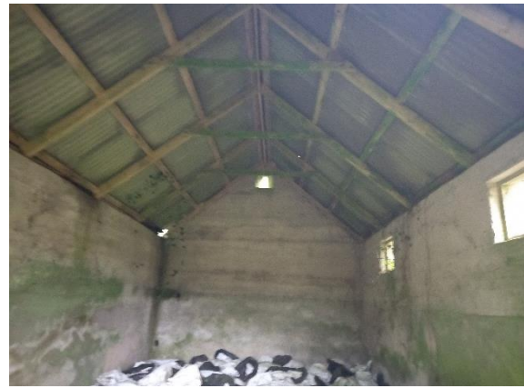
Interior of a building at B_06
